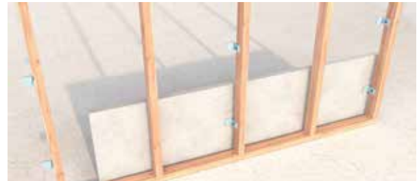
Image 5 – First Panel in place
