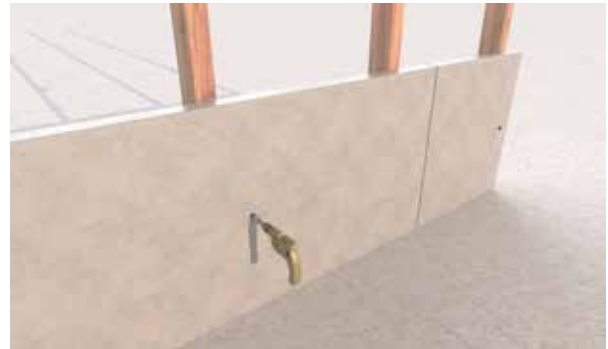
Image 8 – Screw through the panel into the bracket
