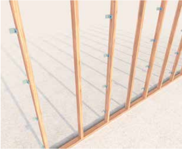
Image 3 – Brackets installed to wall
