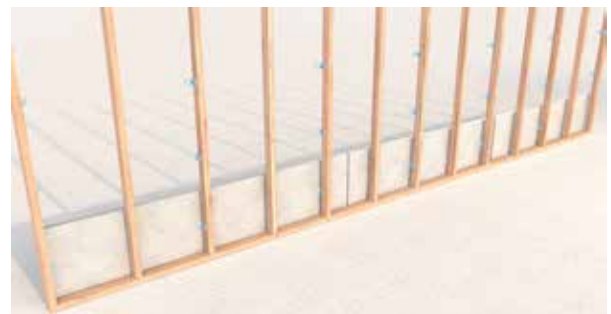
Image 6 – First row of panel installed
