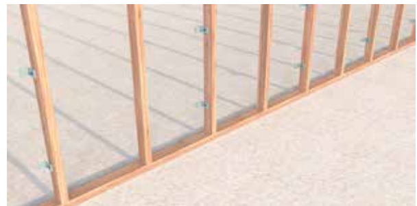
Image 2 – Bottom Row of Brackets installed
