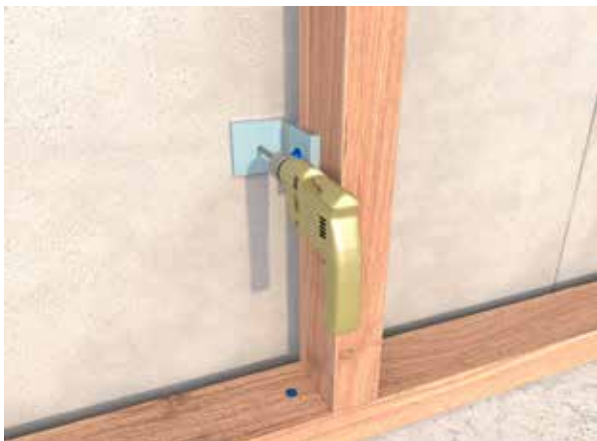
Image 7 – Drill a pilot hole through the panel
