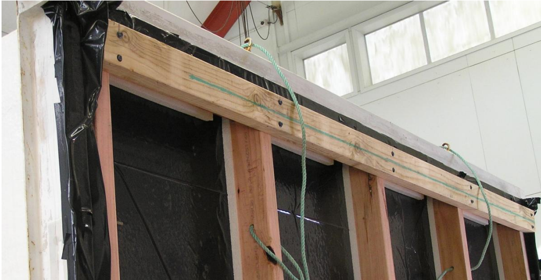
Figure 5. Detail of strong-backs at the top
