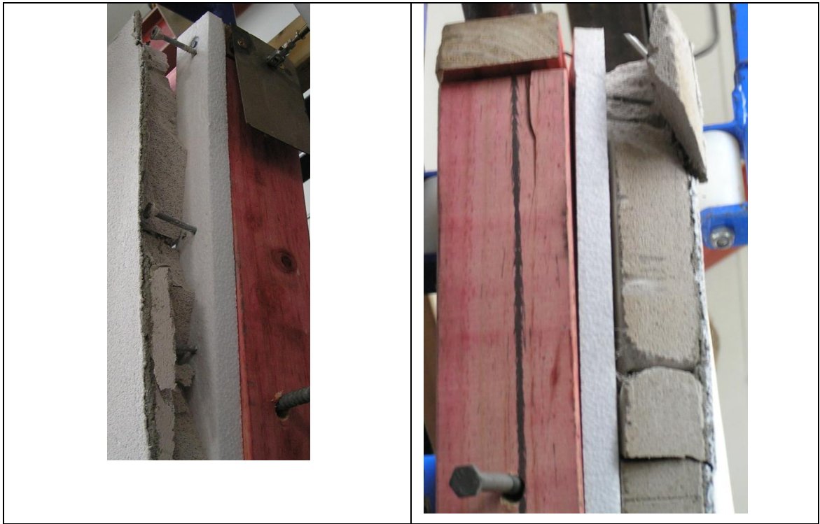
Figure 6. Top of panels at both ends after \pm 55 mm cycling
