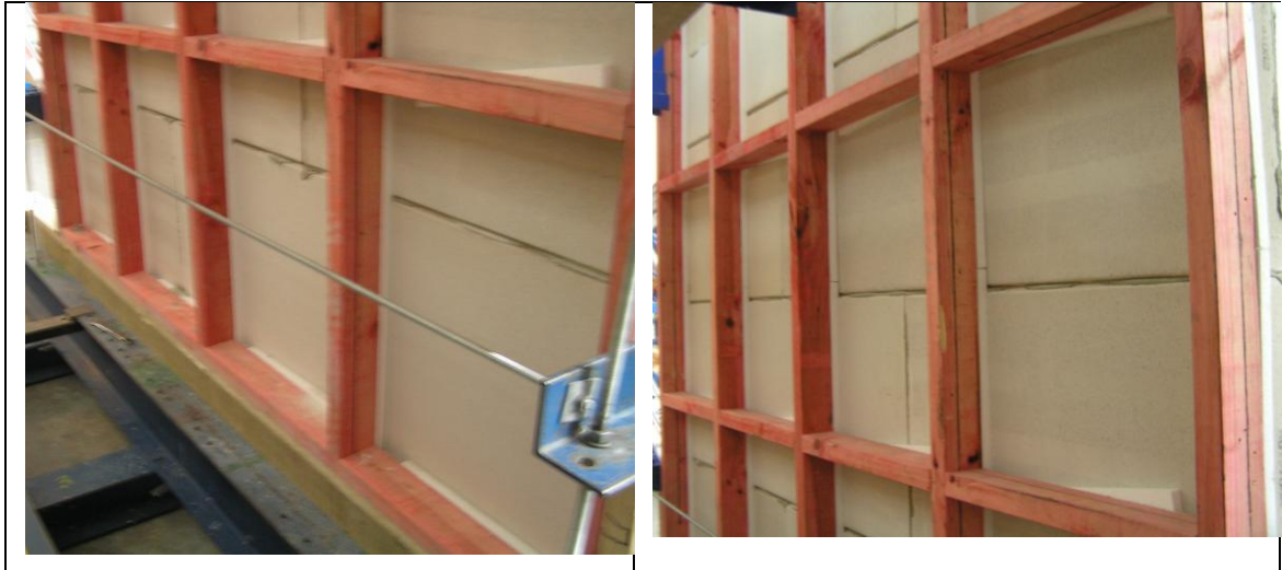
Figure 2. Rear face of wall construction
