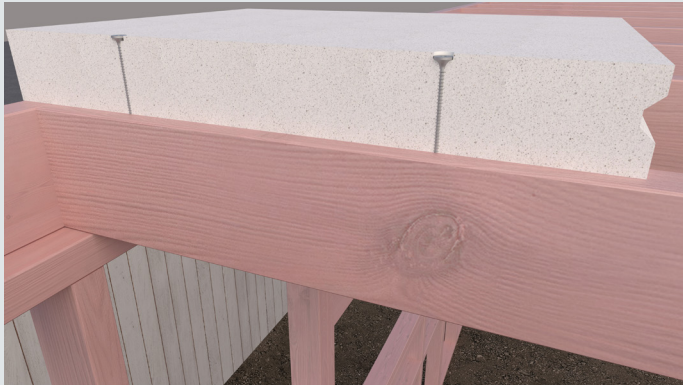
Image 9 – Fix each panel 150mm from the long edges along the joists
