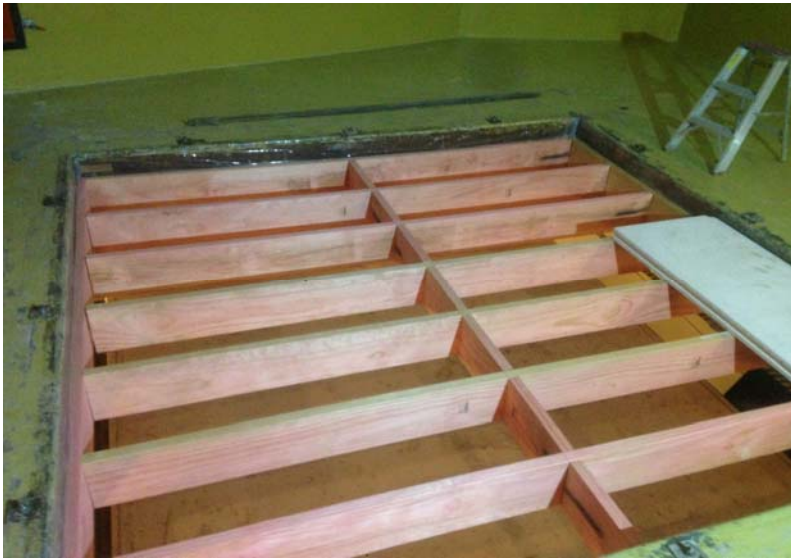
Figure 2: Floor framing showing the central joist nogs
