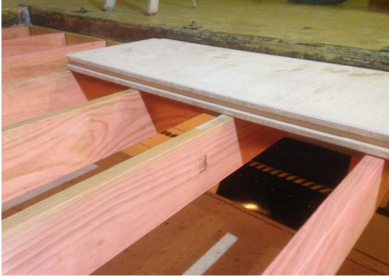
Figure 1: Placing the Rockcote panels on the timber joists
