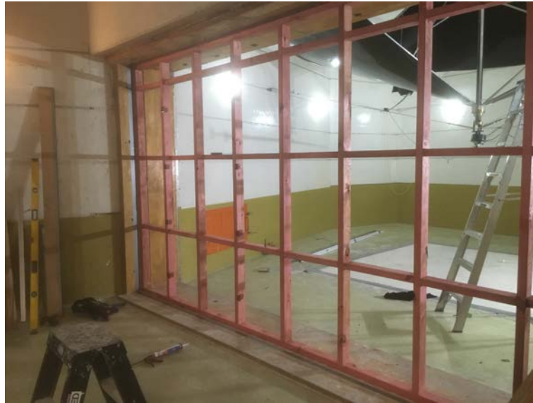
Figure 1.1: 90x45mm studs and nogs
