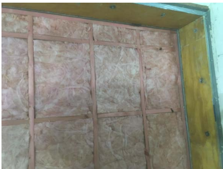
Figure 1.5: Thermal insulation material installed
