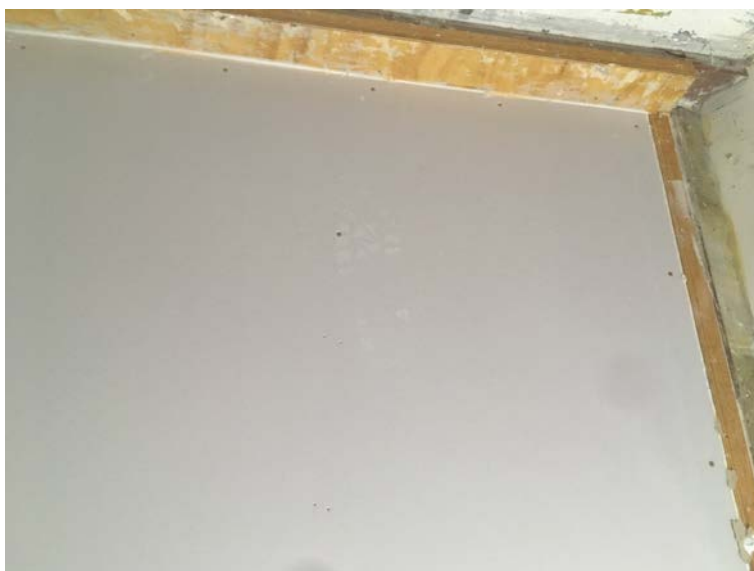
Figure 1.6: Plasterboard applied to wall
