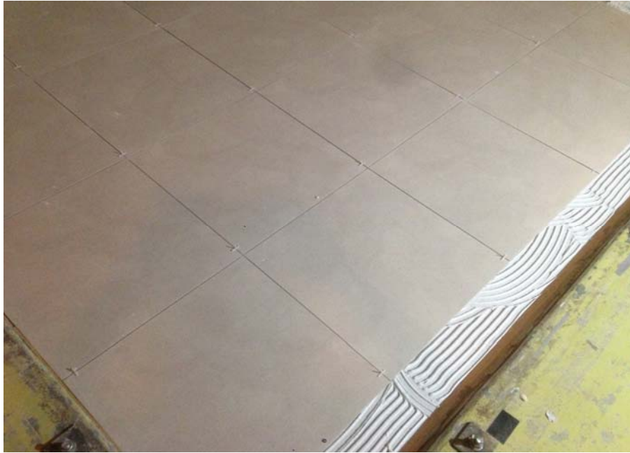
Figure 3: Tiles laid out on test floor
