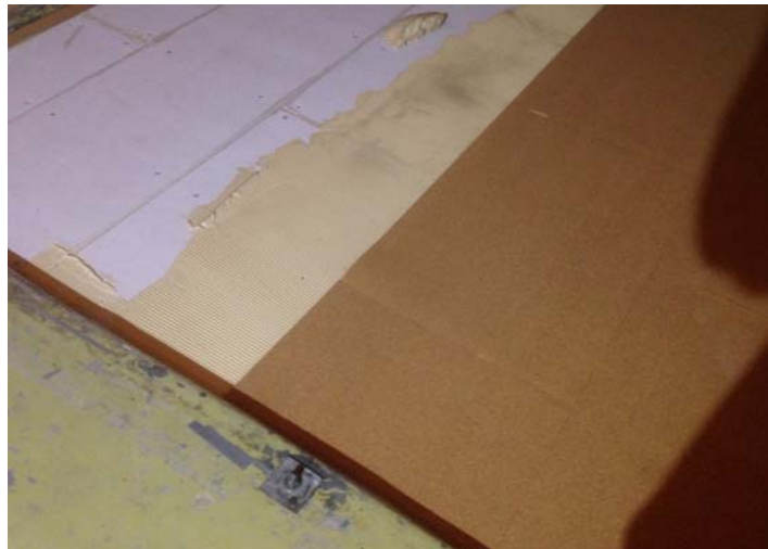
Figure 1: Cork layer being adhered to the original floor surface
