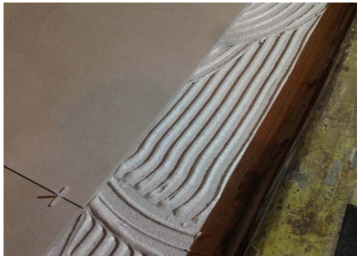
Figure 2: Tiles being adhered to the layer of cork
