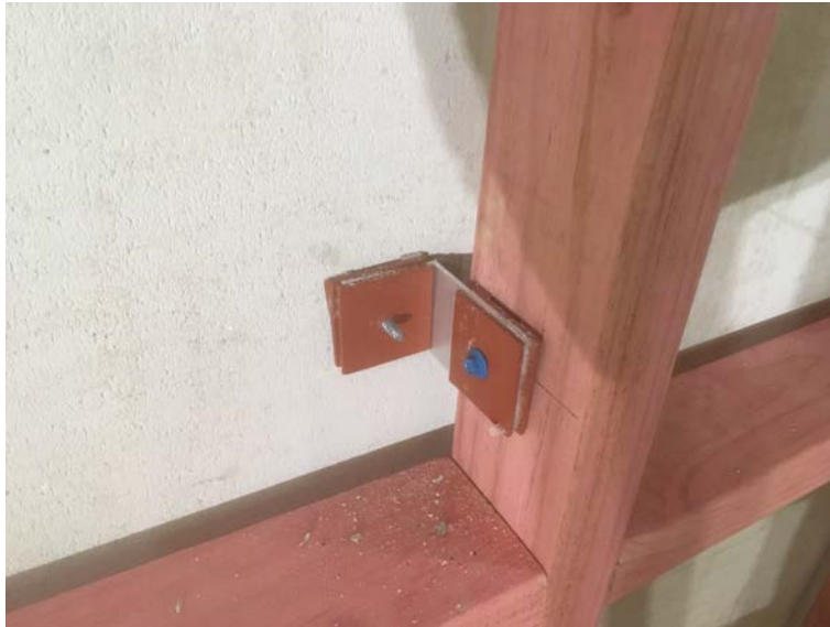
Figure 1.3: Panels fastened to studs
