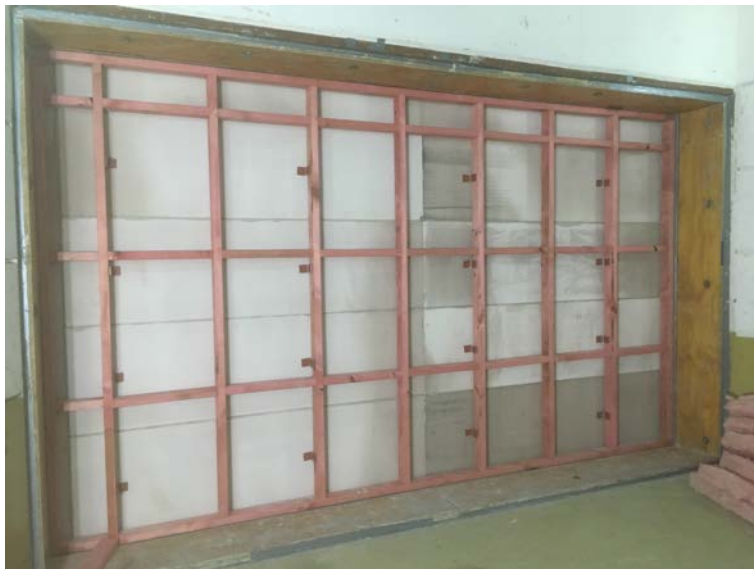
Figure 1.4: Panels installed over the wall
