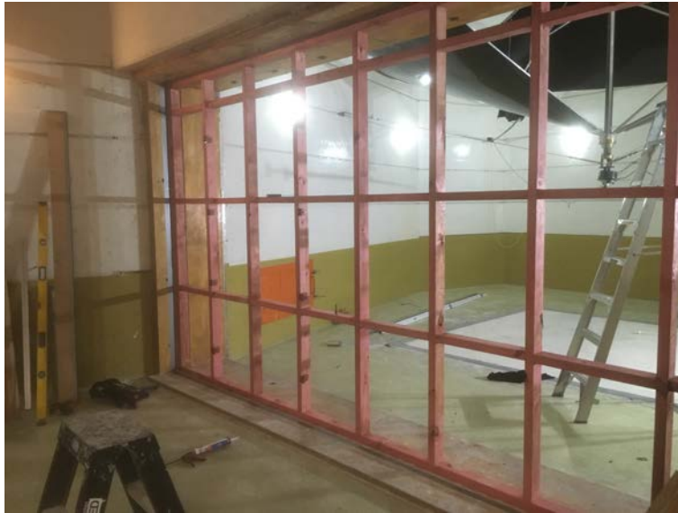
Figure 1.1: 90x45mm studs and nogs
