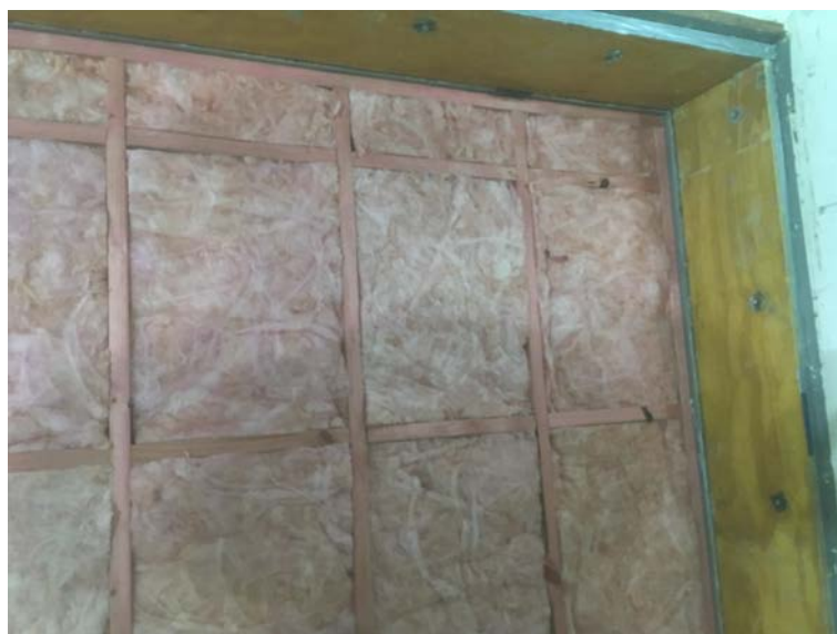
Figure 1.5: Thermal insulation material installed
