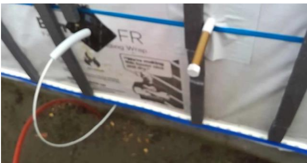
Figure 6: Showing closure drained cavity strip at bottom.
