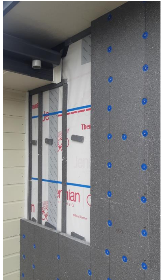
Figure 8: Graphex being installed with plastic washers and nails.
