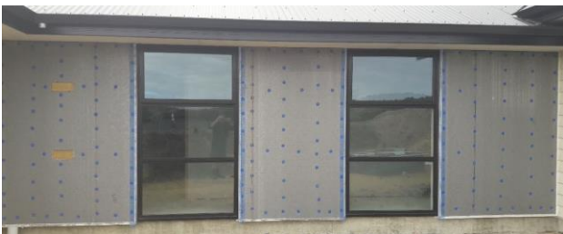
Figure 7: System installed ready for plaster.
