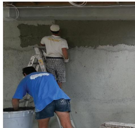
*Existing building strengthened using the Seismolock system*
