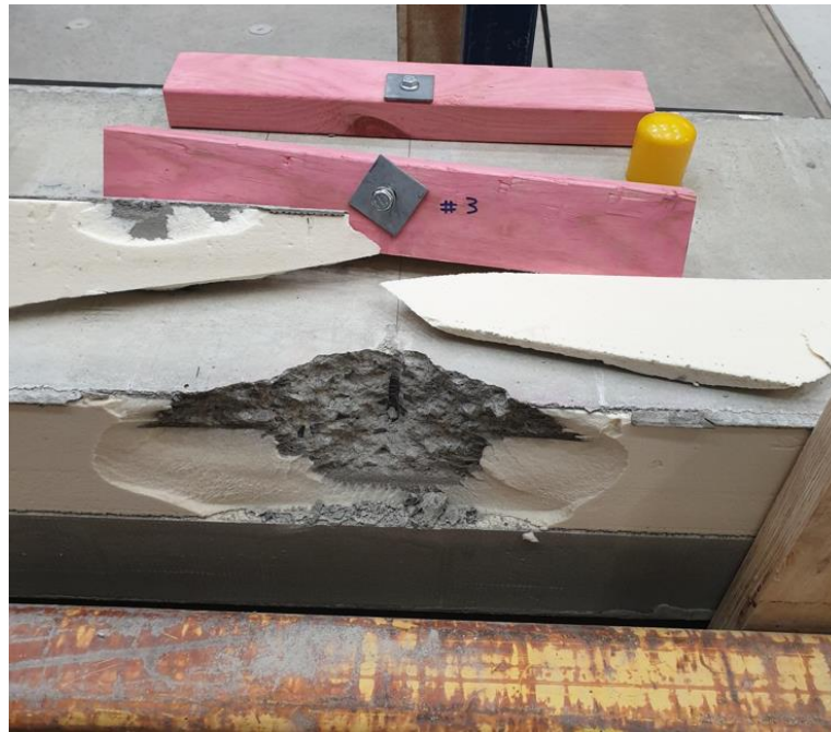
Figure 7. General failure with out-of-plane loading.
