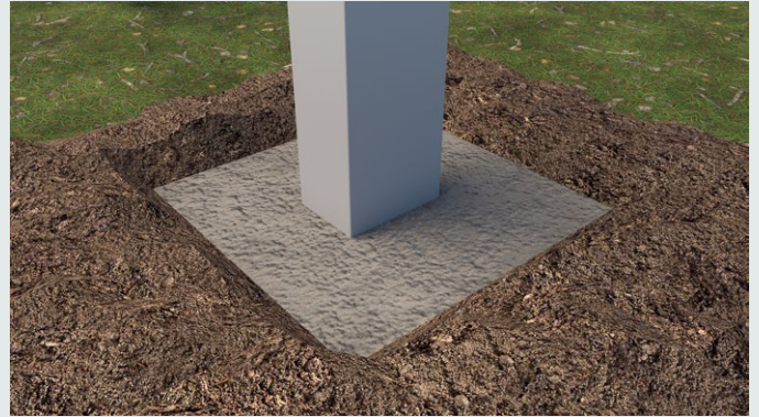
Post installed with concrete poured around it slightly below ground level.
