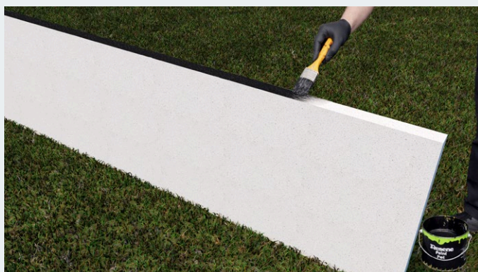
Protecting the bottom panel using Resene Water Lockout.
