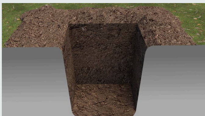
Hole excavated approximately 600mm.
