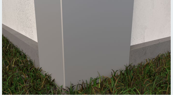
A concrete mowing strip installed against the panel to prevent damage when mowing lawns.
