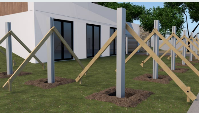
Posts installed into the holes with temporary bracing.
