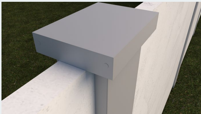
An exposed capping installed to the columns.
